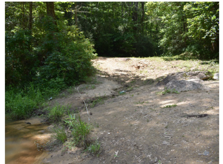
Erosion/rutting channels sediment into the Chauga River from gravel/dirt roads. Photo: Steven Pruitt
