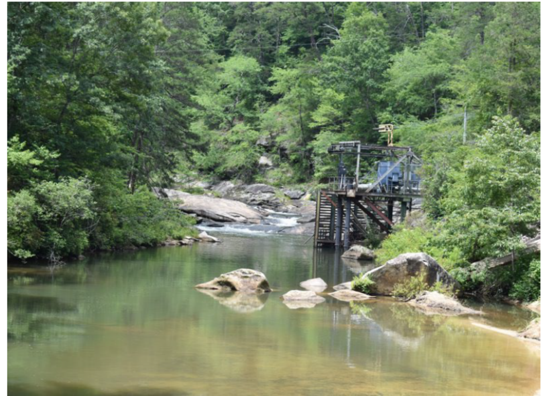
City of Westminster water intake, Chau Ram County Park. Photo: Steven Pruitt
