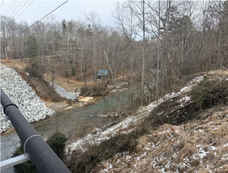
Post-removal of the historic bridge at Hwy 76. Photo: Stu May
