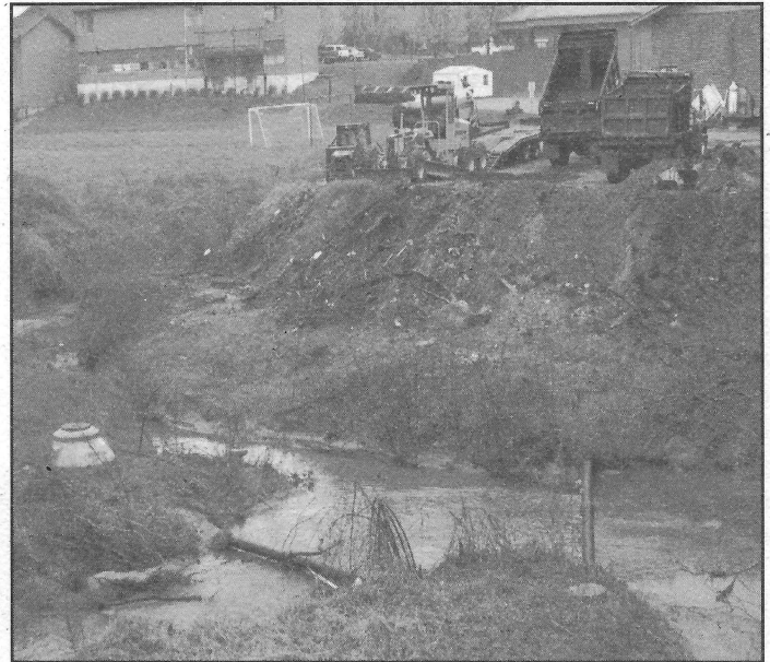
The "arm pit" of the Stekoa Creek watershed: dumping fill in the flood plain; sewage lines in the creek; and, flood-prone manholes. This site is at the crossing of Marsengill & Shadyside St. in Clayton.
