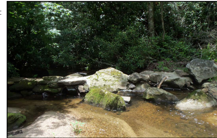
Boulders, large river rocks and plastic culverts were cemented into place across the Chattooga River, creating an illegal and unsightly impoundment located on public lands at the base of Silver Slip Falls.
