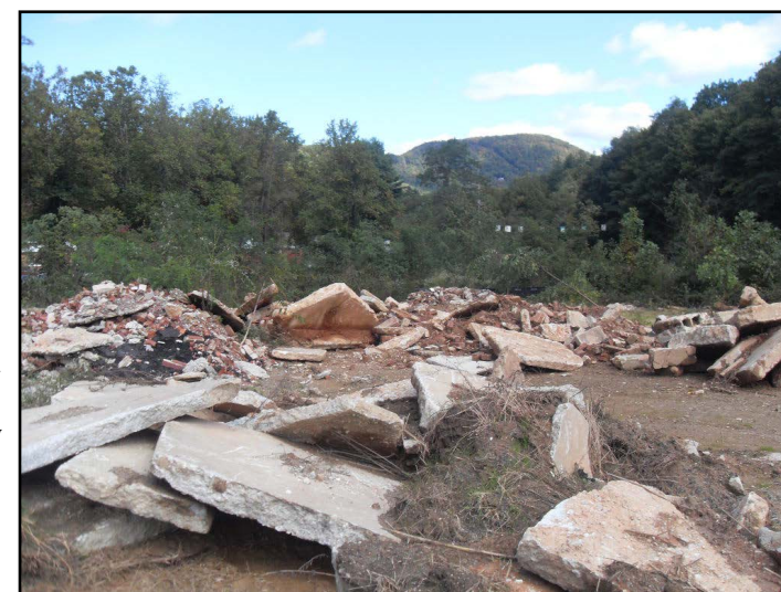
The Stekoa Creek Park site was filled with hunks of concrete as well as overgrown with kudzu, privet and poison ivy.
