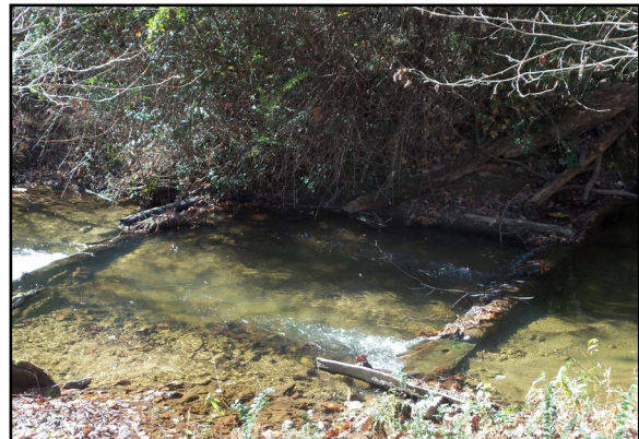
Two large, notched timbers embedded in Stekoa Creek are the remains of the mill pond dam.
