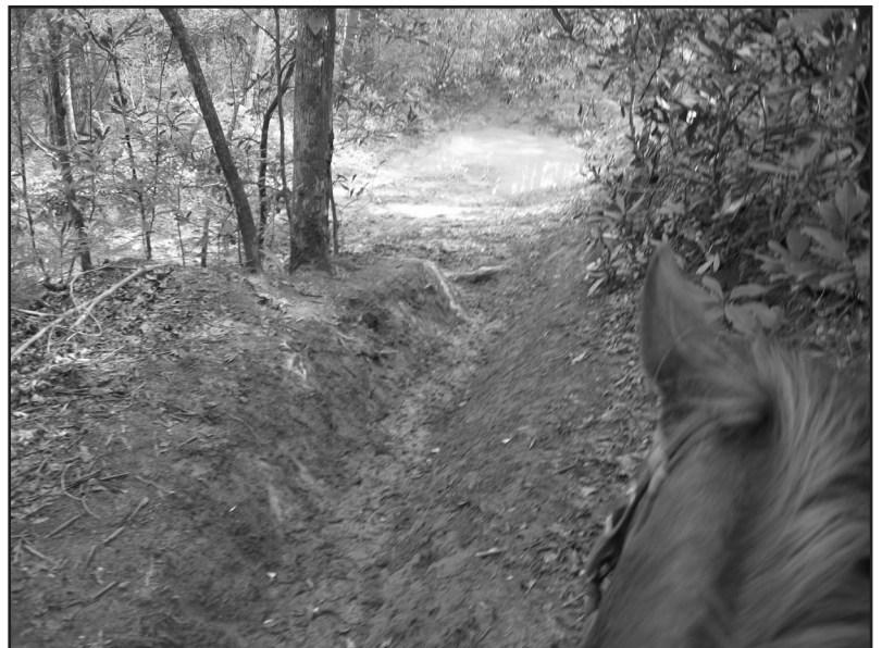
A view from horseback of a section of rutted and eroding horse trail that should be rerouted, near Earls Ford on the GA side of the Chattooga River.
