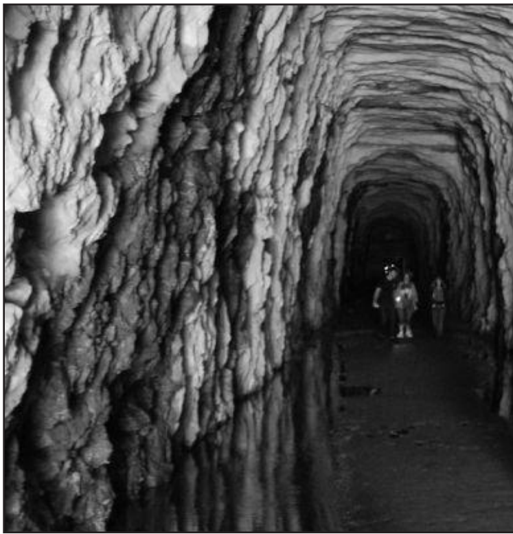
Stumphouse Tunnel in Oconee County, SC, was dug using only hand drills, sledge hammers and black powder. Visitors can explore the tunnel, which is at Stumphouse Tunnel Park on Highway 28 six miles north of Walhalla.
