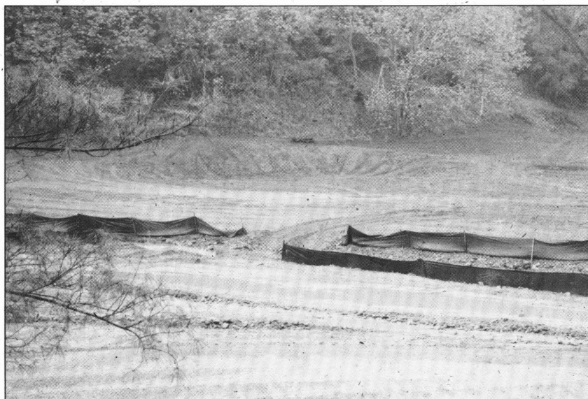
A break in the silt fencing next to the creek was not allowed in the site plan.
