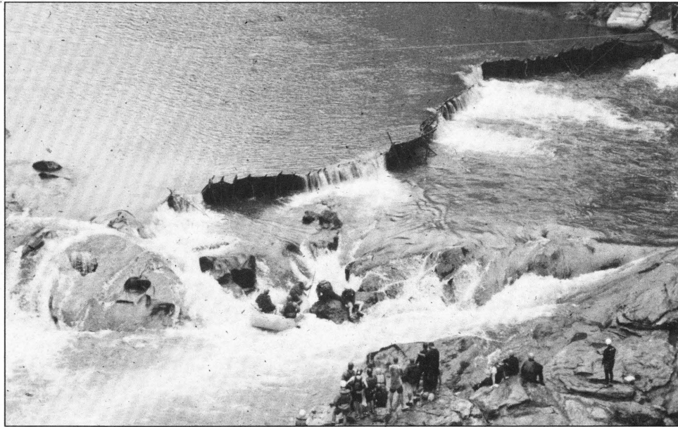
In the first portadam attempt, the river rose behind the dam and breached over it in several places. The dam breached because it was set up to attempt diverting the whole river towards the Georgia side, against its natural flow. Nevertheless, a quick search ensued.
