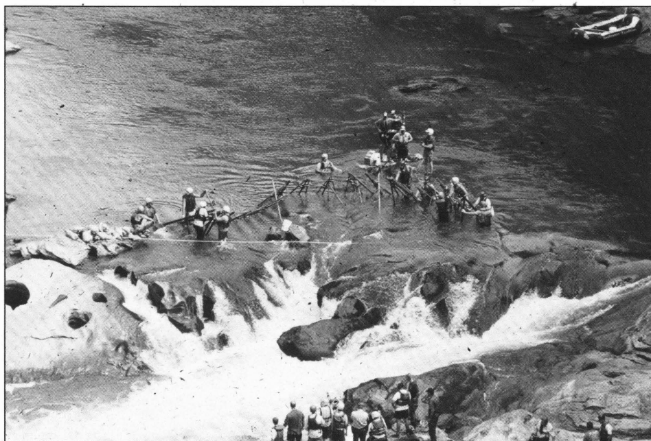
In the second attempt, the frames were placed in a horseshoe fashion, open end downstream, in a tight formation directly above the slot in the middle of the rapid.
