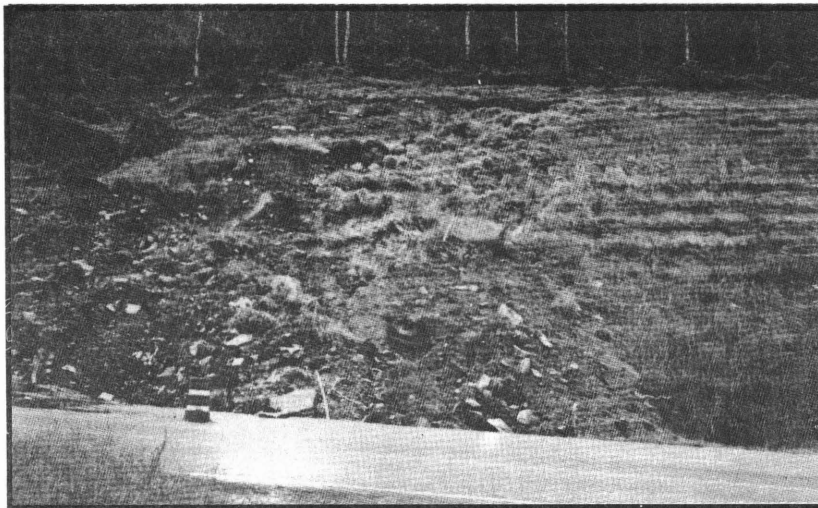
A slumping road cut during reconstruction of Highway 76 near Clayton, GA, impacting Cherchero Creek, a tributary of Stekoa Creek
