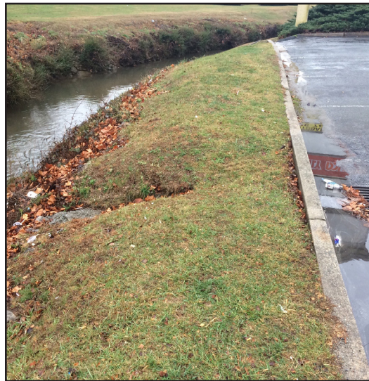
The large parking lot adjacent to Stekoa Creek on Hwy. 441 in Rabun Co. will be modified to stem the flow of polluted stormwater into the creek.
