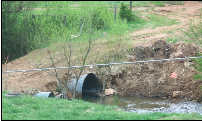
Undersized culverts in Stekoa Creek, installed by way of an agricultural exemption, have created eroding stream banks.
