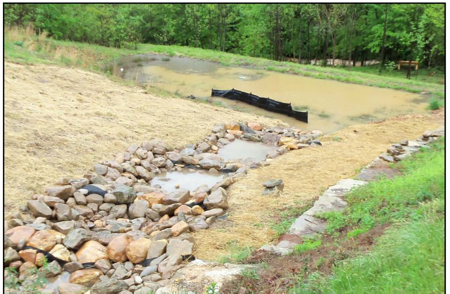
A rain garden constructed at Stekoa Creek Park in 2014 prevents polluted stormwater from Highway 441 from flowing into Stekoa Creek.
