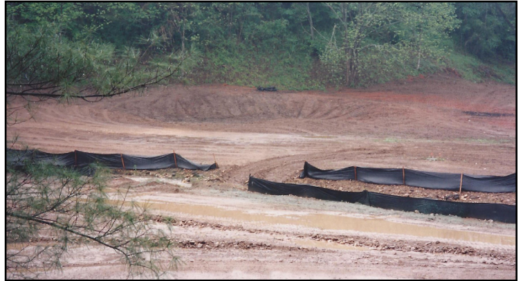
The absence or improper design of BMPs during reconstruction of the Kingwood golf course caused a massive amount of dirt to wash into Chechero Creek, evidence of which remains today.
