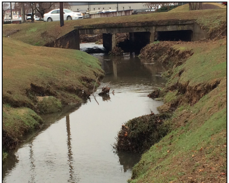
Stekoa Creek's streambanks exhibit severe erosion damage from the impact of relentless stormwater runoff from Hwy. 441 and parking lots that cover the creek's 50-foot buffer zone.
