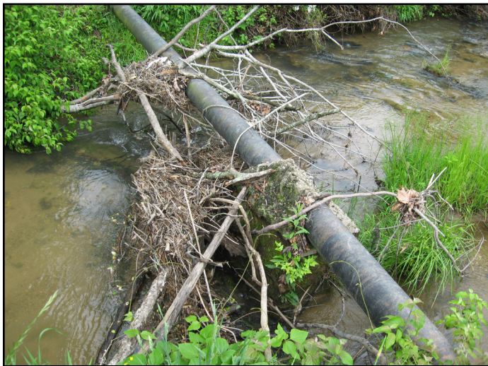
Sewage lines cross Scott Creek, which often leads to flotsam and debris jams on the infrasturcture.
