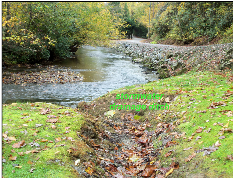
Stormwater discharge from Rickman Airfield Road is directed into Stekoa Creek through ditches and culverts.
