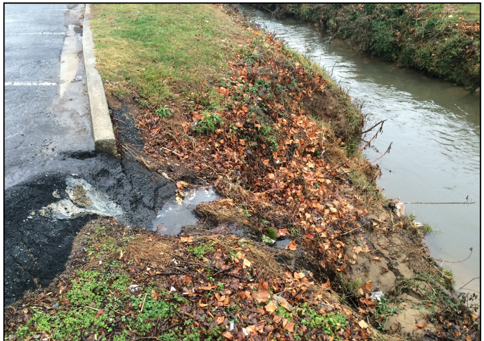
A large parking lot built in the flood plain next to Stekoa Creek covers the stream's 50-foot buffer zone, and discharges all of its stormwater runoff directly into the creek.
