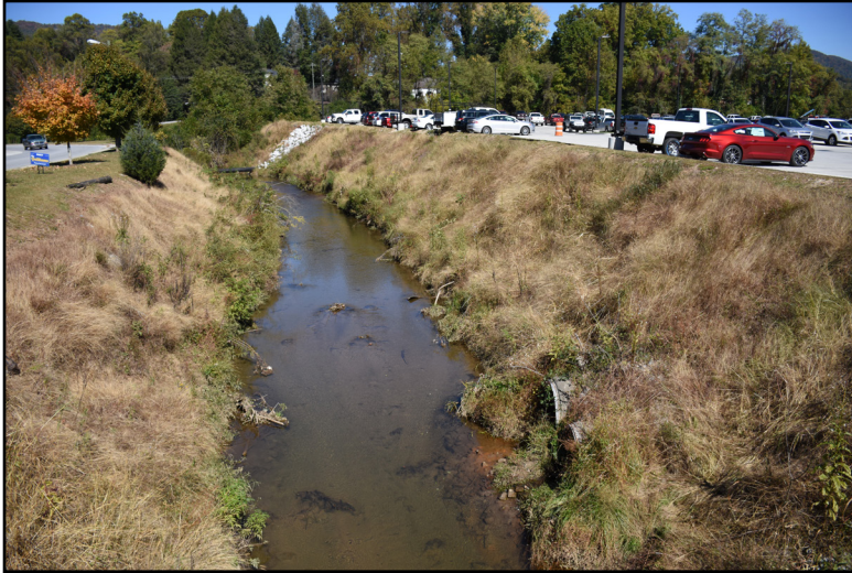
Sections of Stekoa Creek in Clayton have undergone hydromodification that includes channelizing and confining the stream within rip-rap embankments.
