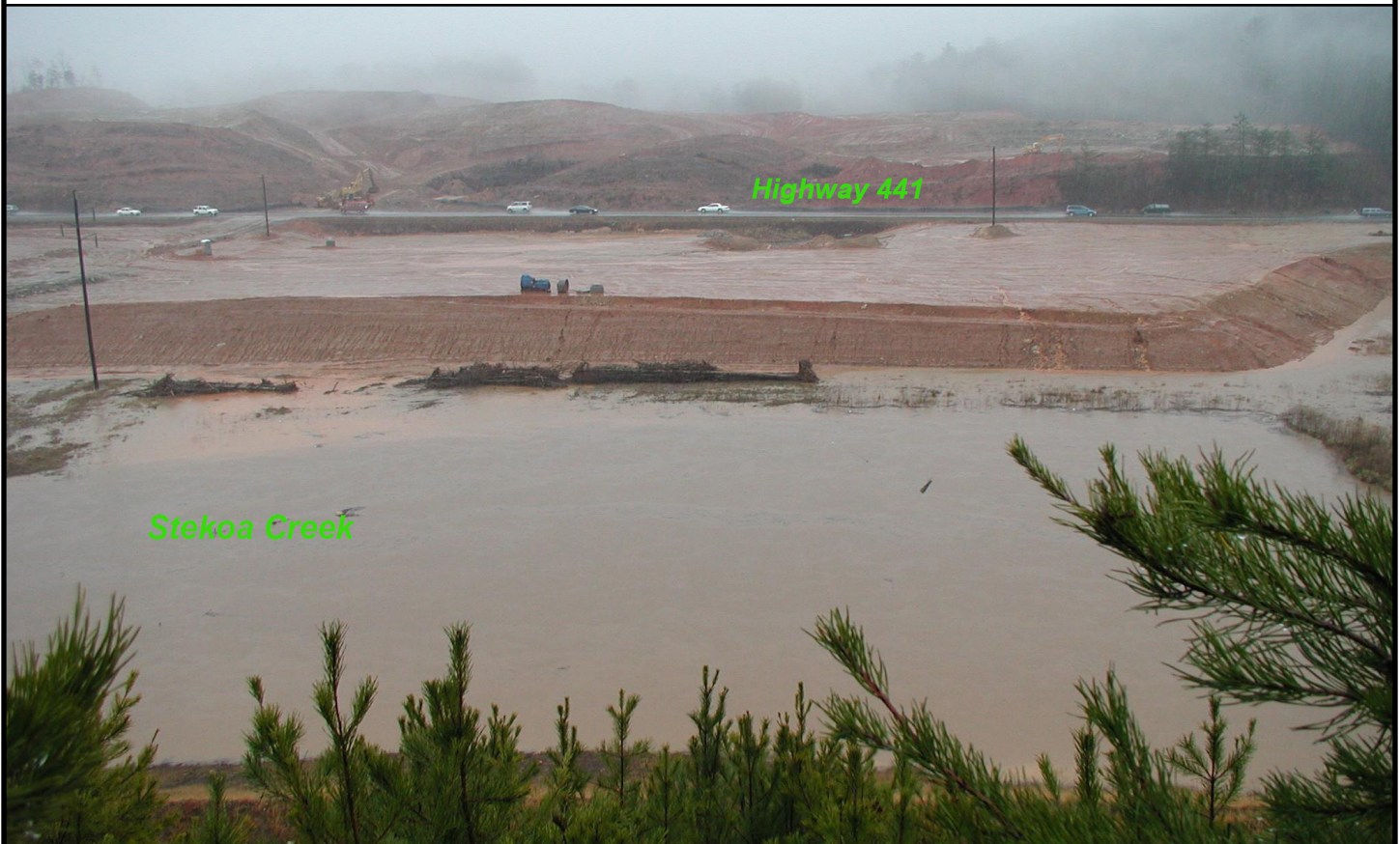
In 2004, the steep topography on the east side of Highway 441 was leveled to make a flat spot for development, and the earth was used for filling a portion of Stekoa Creek’s floodplain, putting a massive amount of dirt into the creek.
