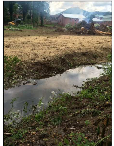
Ginger Creek, tributary to Scott Creek, exhibits a lack of BMPs in its stream buffer zone as illustrated by this recent (5/2015) clearing operation.
